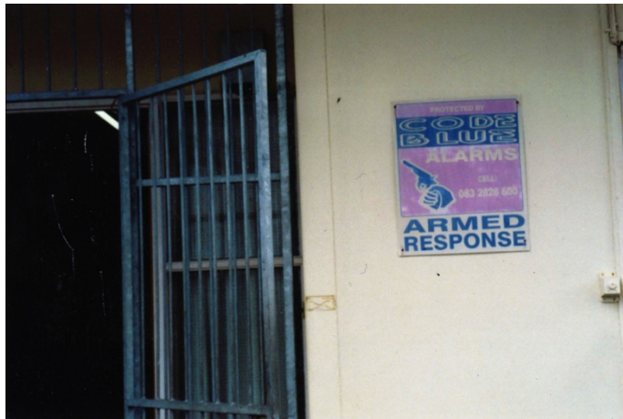
Figure 2 Pefferville Entrance Before Renovation
